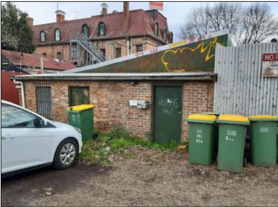
Figure 6 Common parking area facing North (closer)
